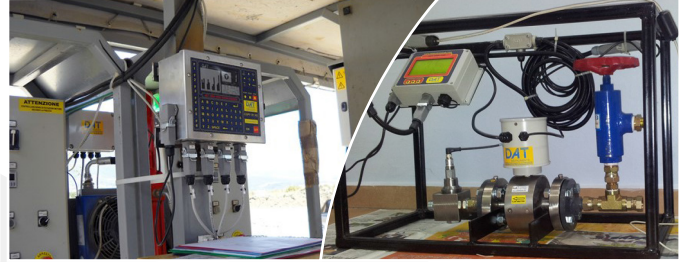
GROUTING, CEMENT INJECTIONS GROUTING, ÇİMENTO ENJEKSİYONU
